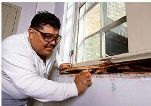
Local or spot treatment with pesticides involves drilling and injecting pesticides into infested timbers, as well as the topical application of toxic chemicals. The electric-current method involves delivering electric energy to targeted infestations. For the extreme cold method, liquid nitrogen is pumped into wall voids adjacent to suspected infestation sites, reducing the area to -20° F. The localized heat method involves heating infested structural timbers to 120° F. The microwave
